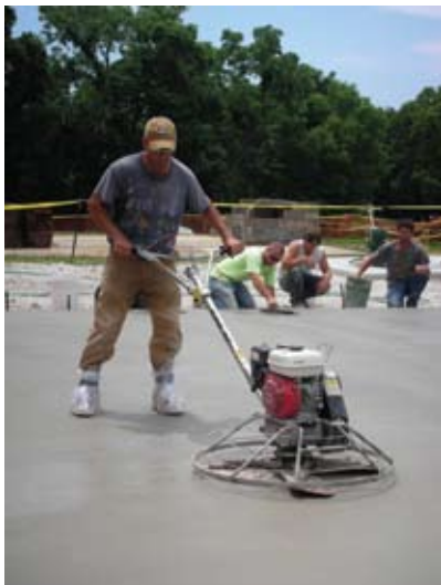
Use of Power Trowel - Year 3
