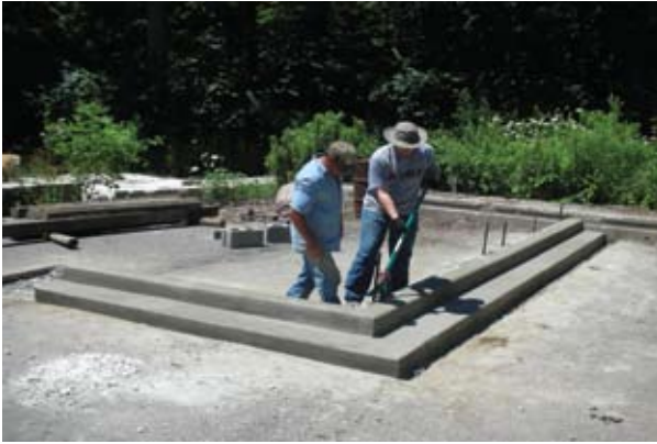
High back curb - Year 2
