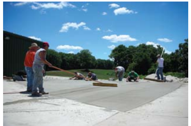
Concrete Slab - Year 2
